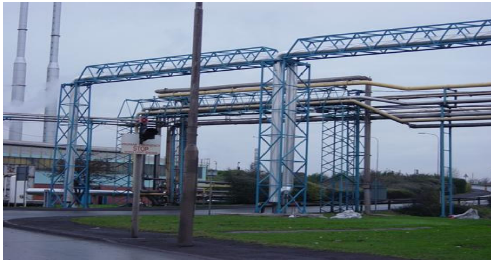
Figure 1: Steam main bridge at Corus
